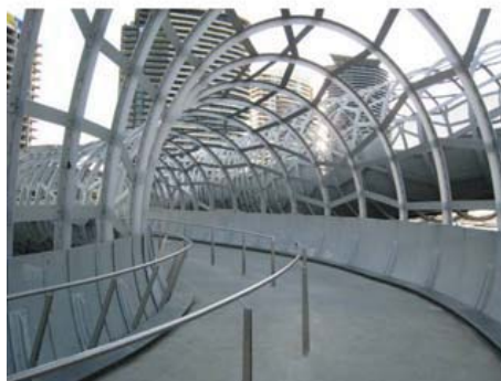
Melbourne, Australia—The bridge provides a moderate level of texture and visual variety. This is interesting enough for pedestrians but better scaled for cyclists.
